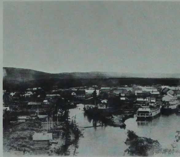
Chena as it appeared during the early part of the century. Located 7 miles southwest of Fairbanks, the area is now a campground.
